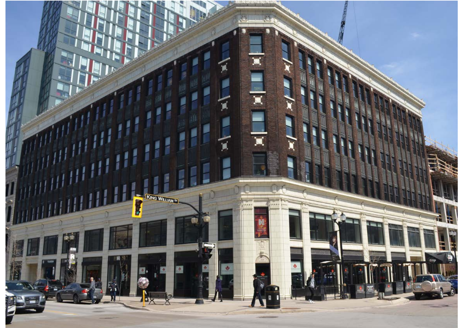
Lister Block with the 20-storey student housing complex behind in downtown Hamilton.
